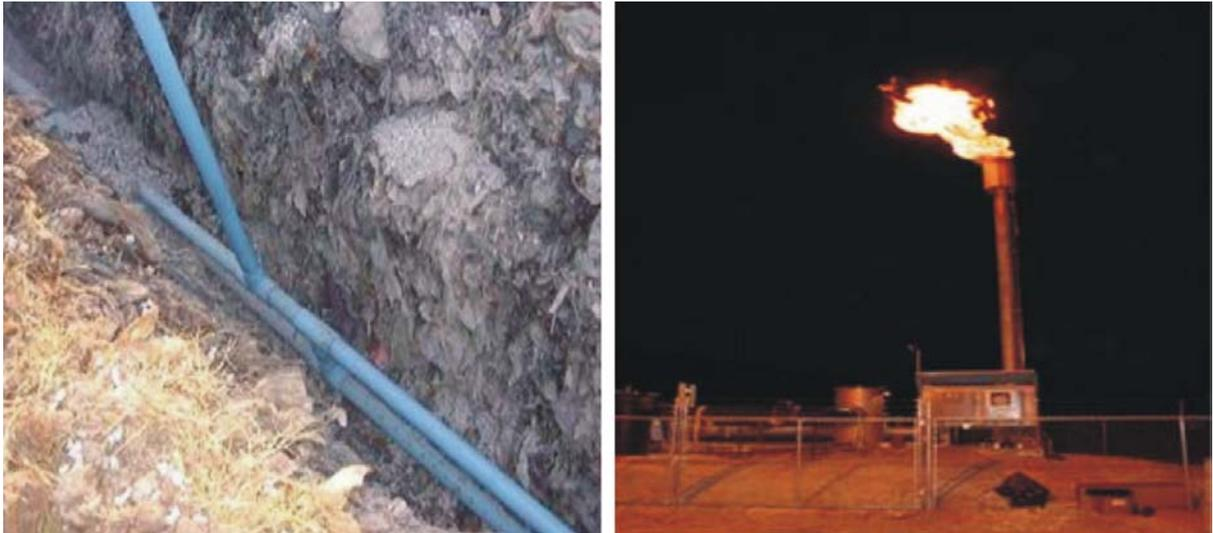
**Figure 4. LFG collection and flaring system**
